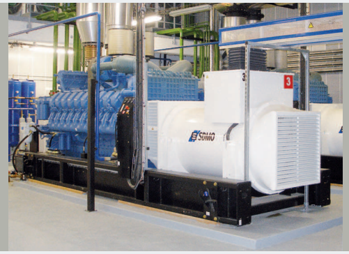
Strip bearing of a cogeneration plant
