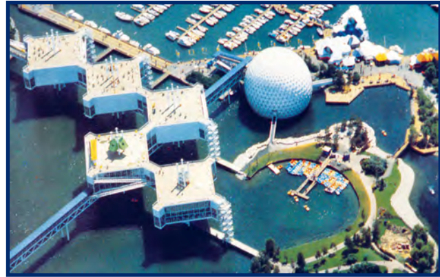
Ontario Place: A Lexcan EPDM Roof installed in 1968
