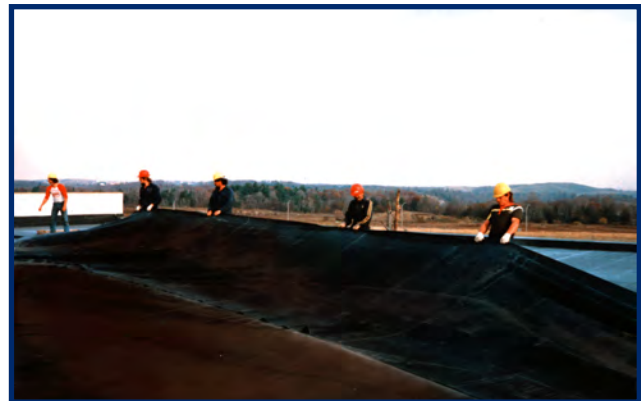
Unrolling Standard EPDM Membrane Sheet
