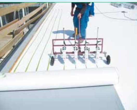
applying the roof sheet adhesive
